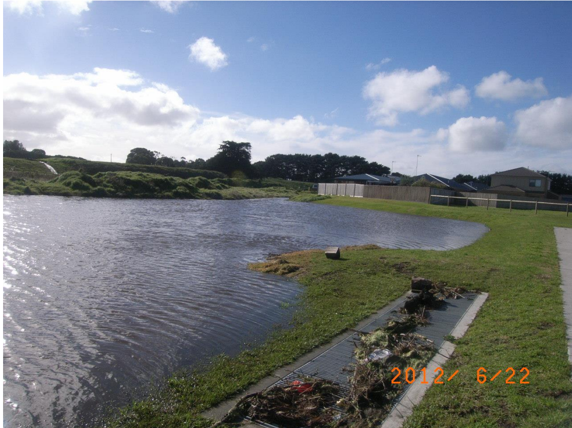
Figure 7.17: The Wreck Creek retarding basin
