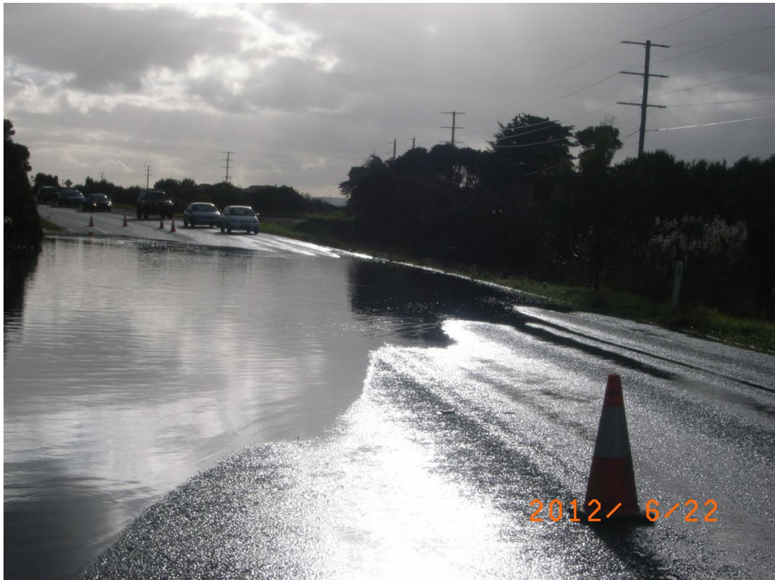
Figure 6.24: Bass Highway flood 22/6/2012
