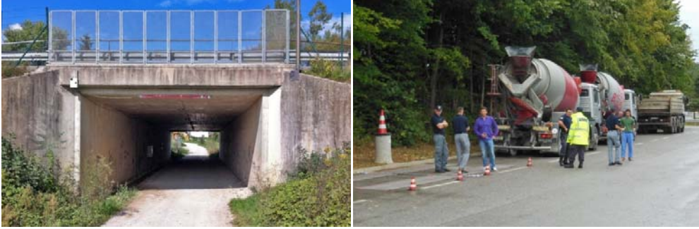
Figure 6: The instrumented underpass (left), and the static weighing of vehicles (right).
