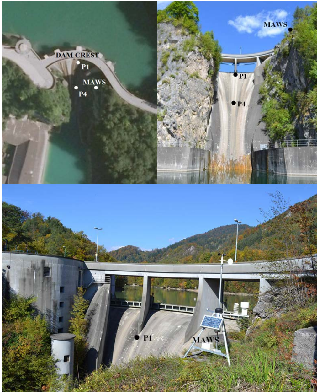
Fig. 3. Location of the MAWS, close to the dam
