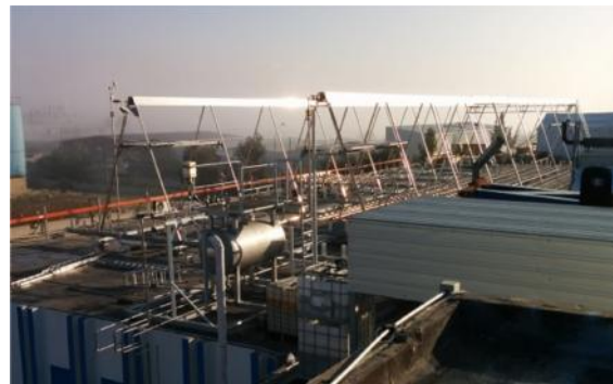
Figure 2 The solar-DSG plant under construction in Jordan - Photo from December 2014
