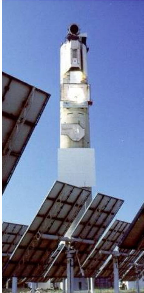
Solar Power Tower
