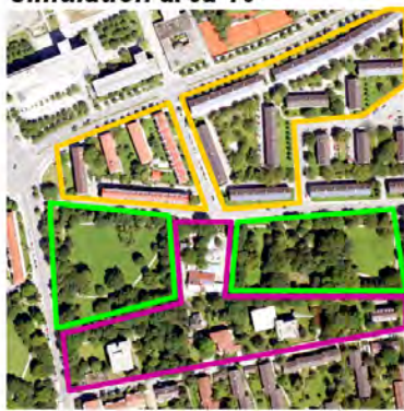
3K aerial photograph
