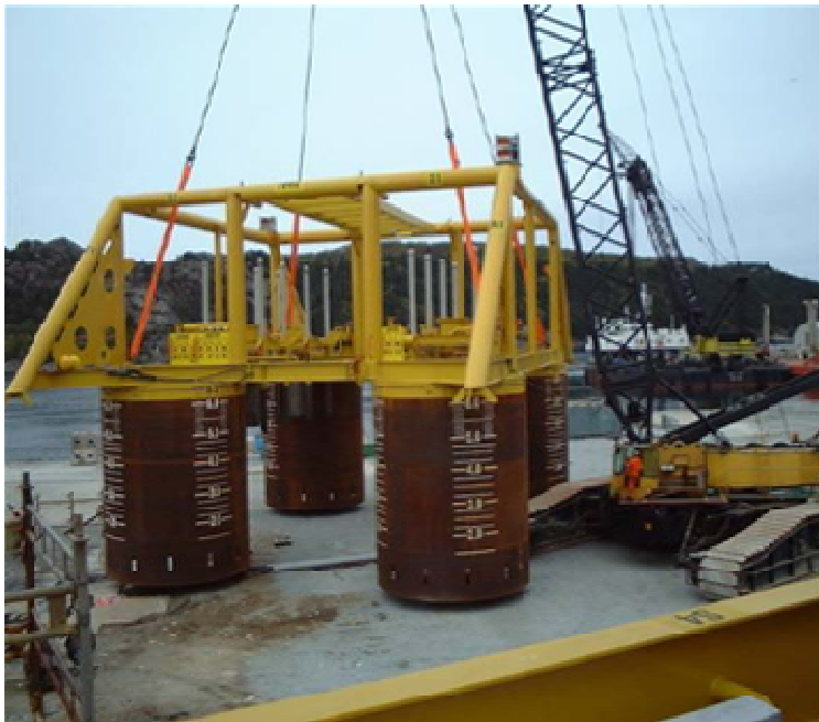
Figure 4.4.b. Subsea template at Kristin Field. (Nergaard, 2008)
