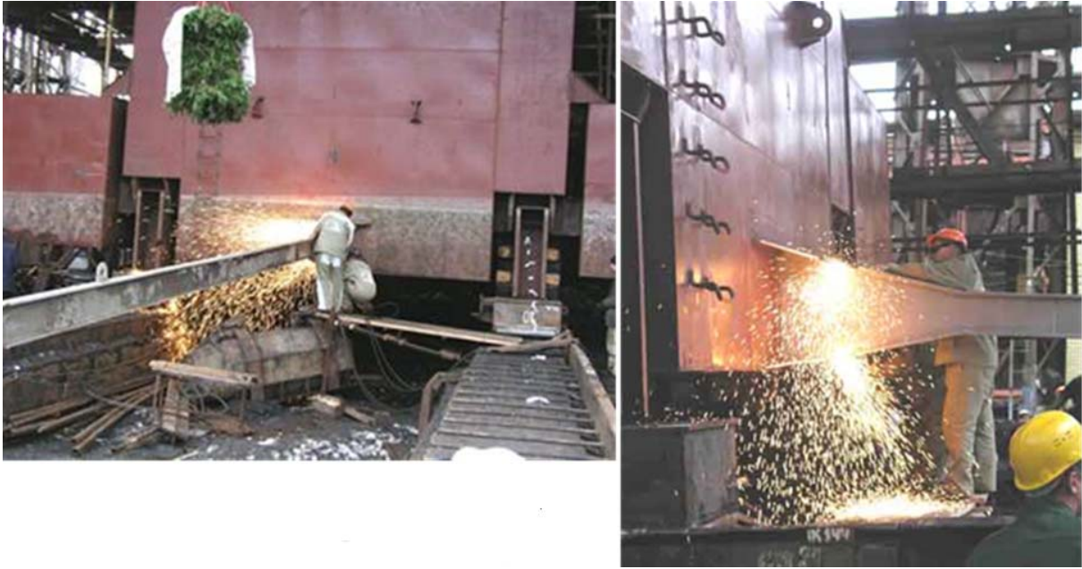
Figure 7.13. Cutting of the vessel's supports.
