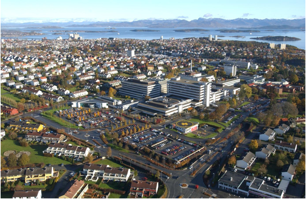
Figure 8. Stavanger University Hospital (Until 2005 Rogaland Central Hospital).
