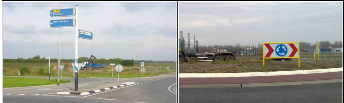
Figure 72: Signposting at the splitter island and traffic sign on the central island
