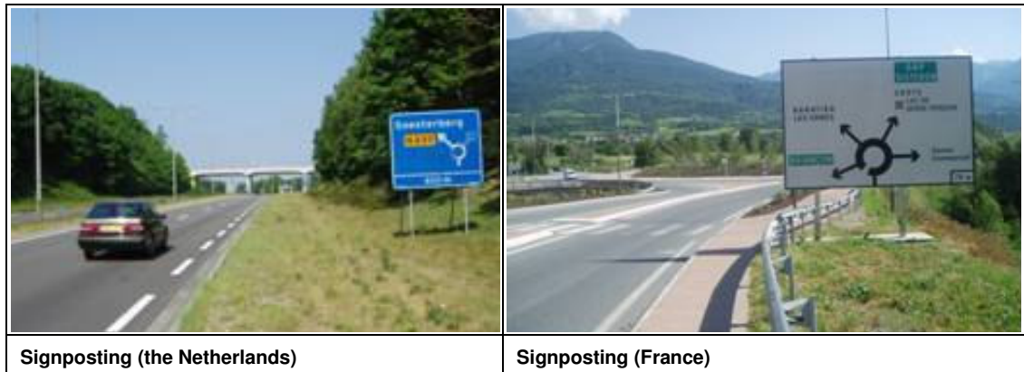
Figure 35: Signposting in advance of the roundabout
