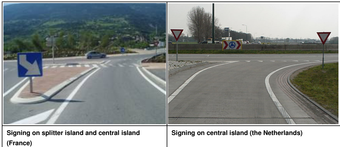
Figure 36: Give way signs on both sides of entry
