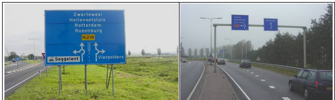
Figure 71: Signposting at 400 meters ahead of the roundabout
