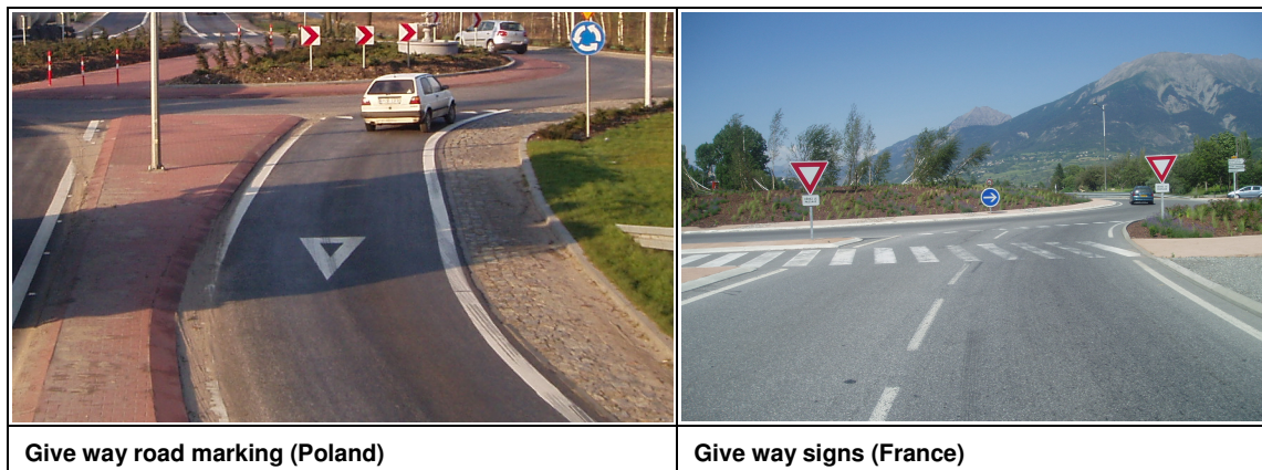
Figure 34: Give way road marking and signs
