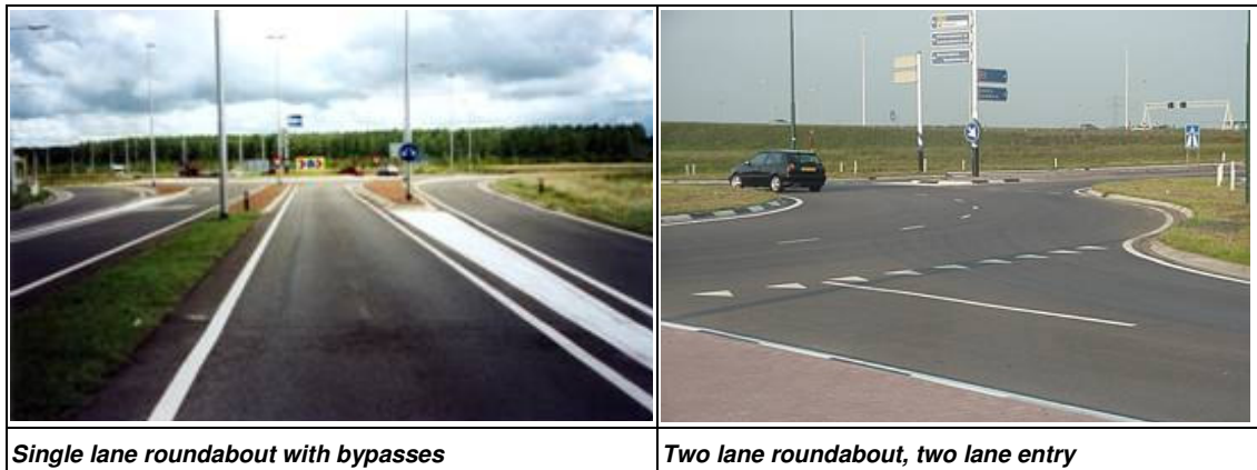
Figure 7: Examples of single and two lane roundabout
