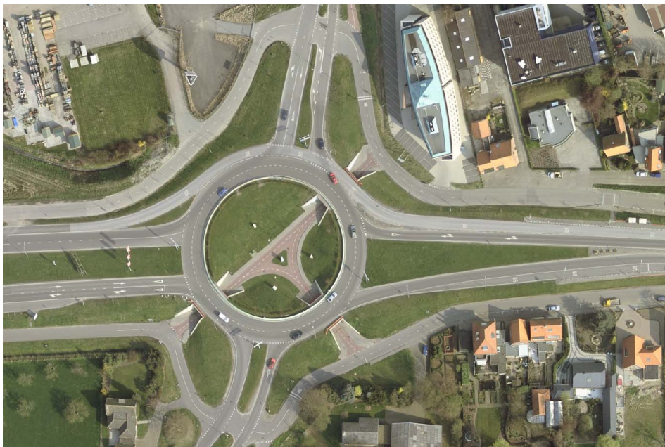
Figure 45: Example bicycle underpasses at a roundabout (the Netherlands)
