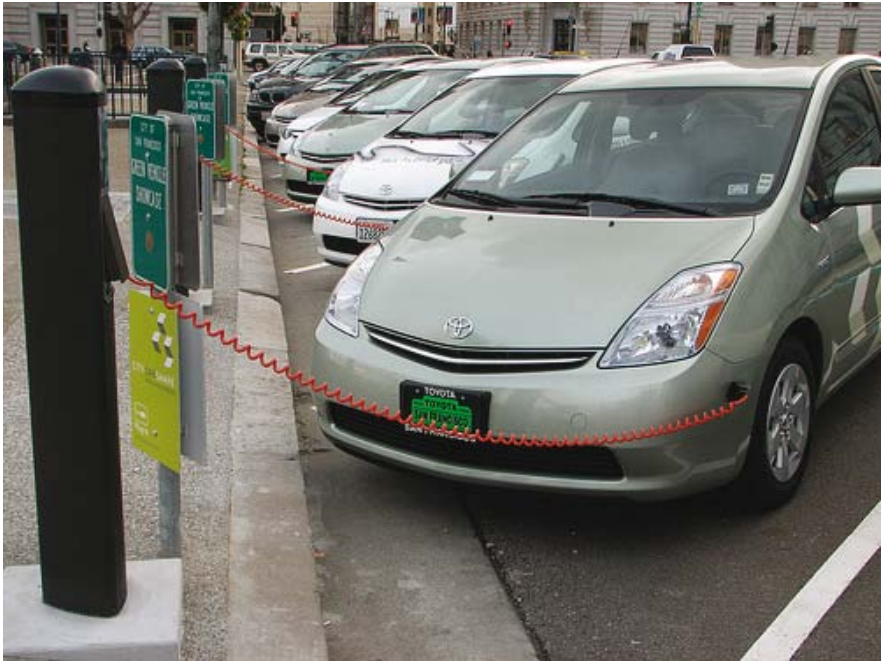
Infrastructure for green transport - plug-in points for hybrid cars in San Francisco. Image courtesy of CalCars.org.
