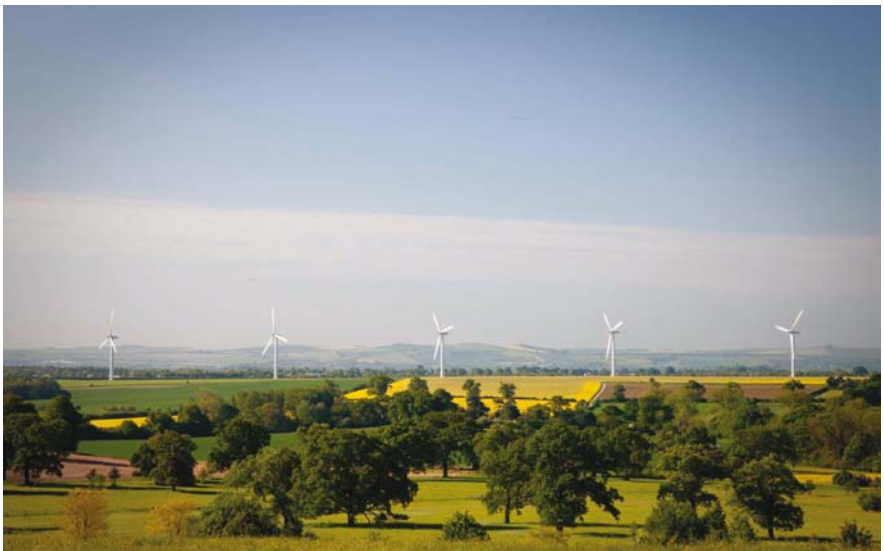
Here is one of Britain's few co-operatively owned wind farms at Westmill in Oxfordshire. It has 2,400 shareholders. Image courtesy of Andrew Watson.
