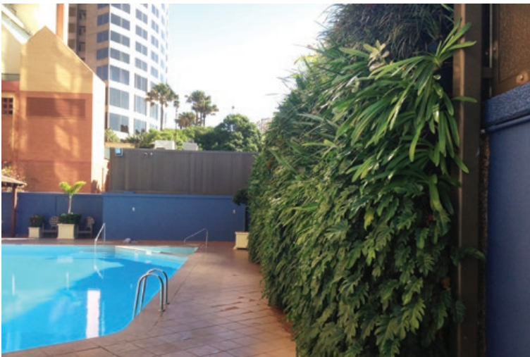
Green wall at Four Seasons Hotel, The Rocks, Sydney.
