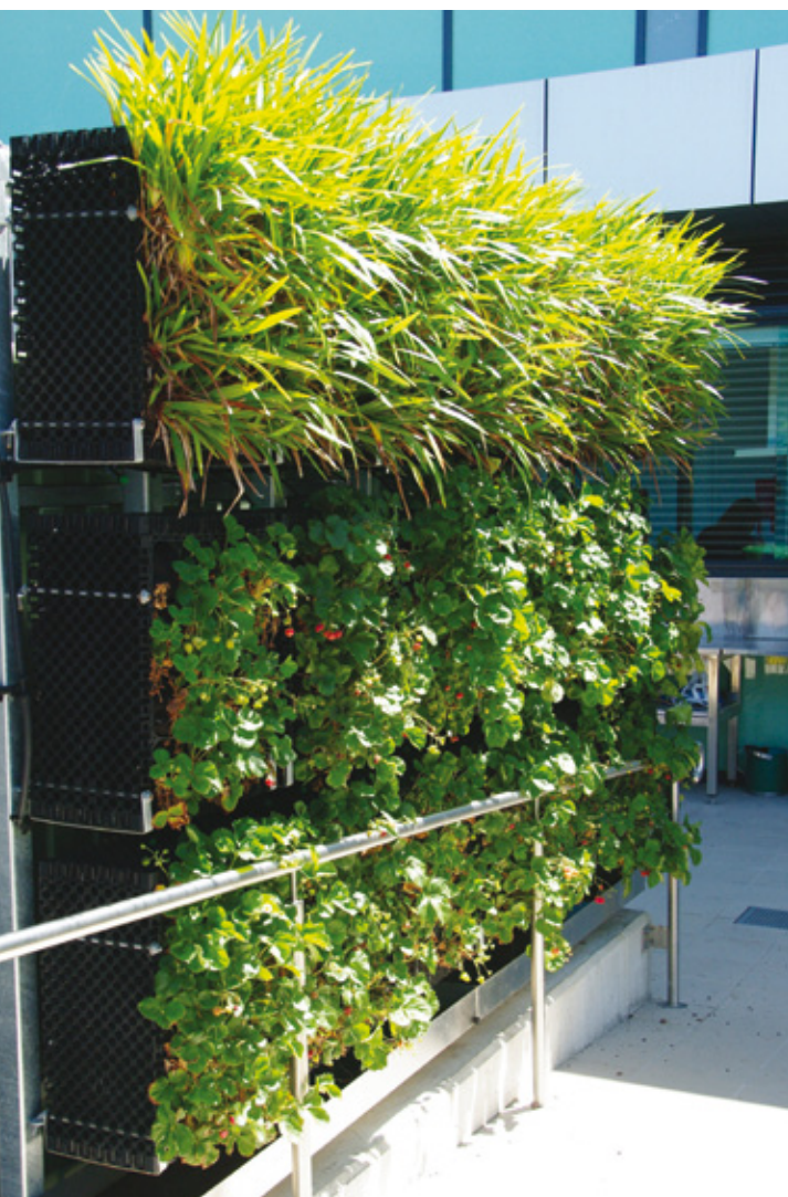
This green wall on the roof of a health care centre in Marion, South Australia, incorporates an inbuilt water tank to provide water supply and structural integrity for double sided modular wall systems, with plantings including strawberries and herbs. Image: Fifth Creek Studio
