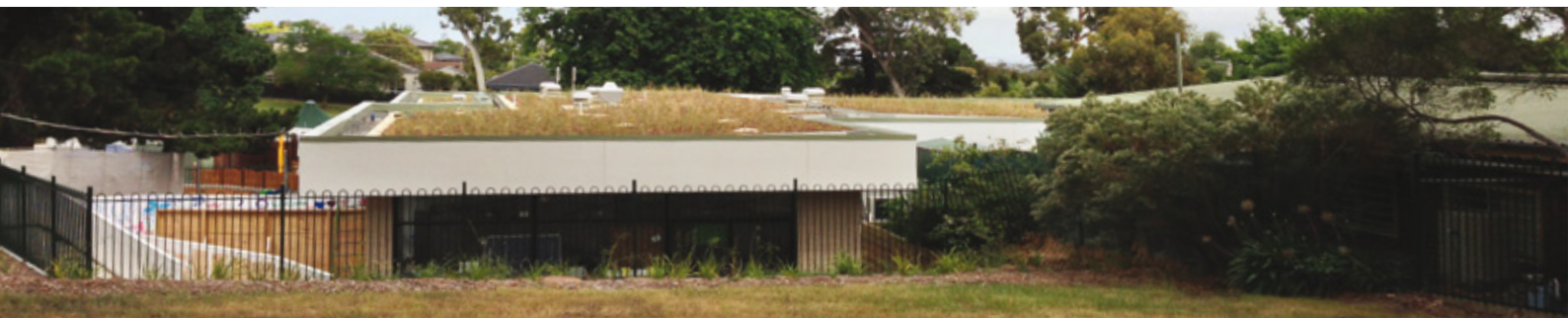
The building sits low in a park, meaning the roof can be easily viewed from street level
