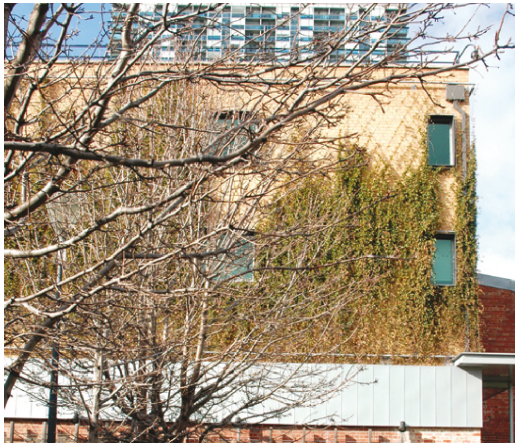
The green facade is now a key element of the view from the University Lawn Precinct
