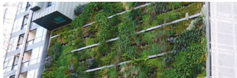
Fytogreen design uses wind tolerant species to shield others on the green wall at the Triptych Apartments, Southbank
