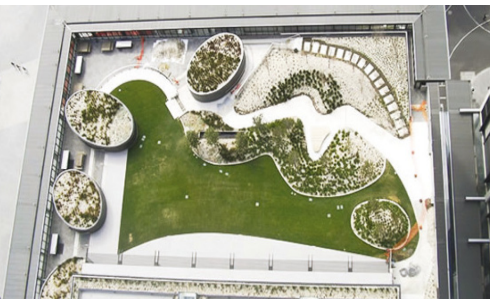
Aerial view of the Freshwater Place green roof after construction
