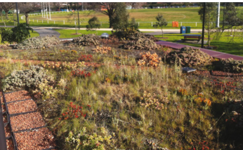
Mixed plantings and non-vegetated zones on The Venny roof
