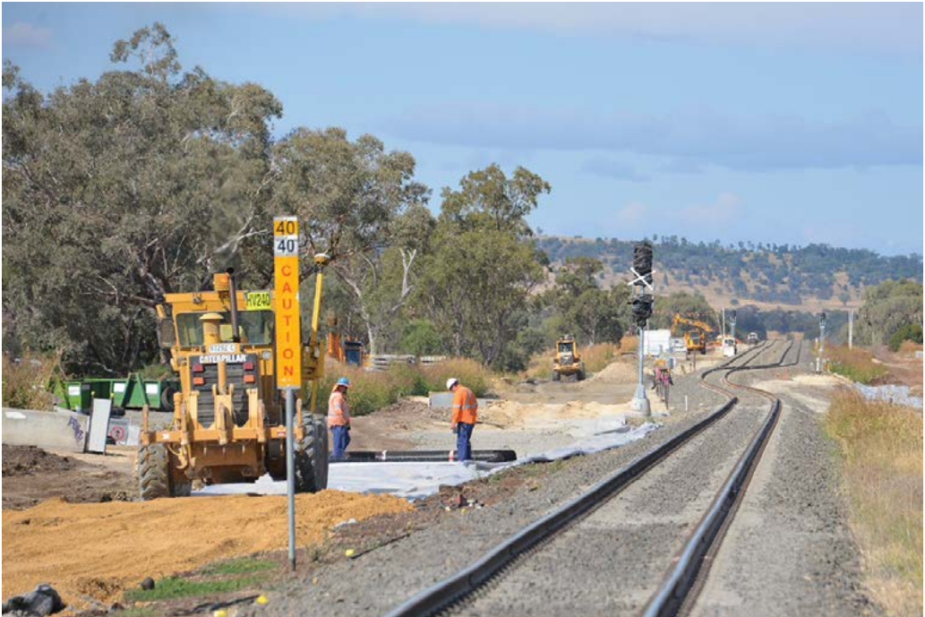
Figure 7 Track capacity expansion, Watermark, NSW
