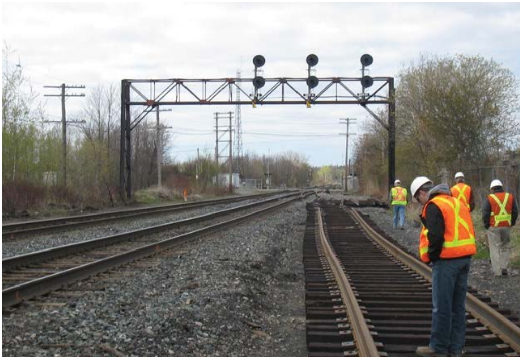
Figure 37 Adding capacity: a third-main line being added near Kingston, Ontario, 2010
