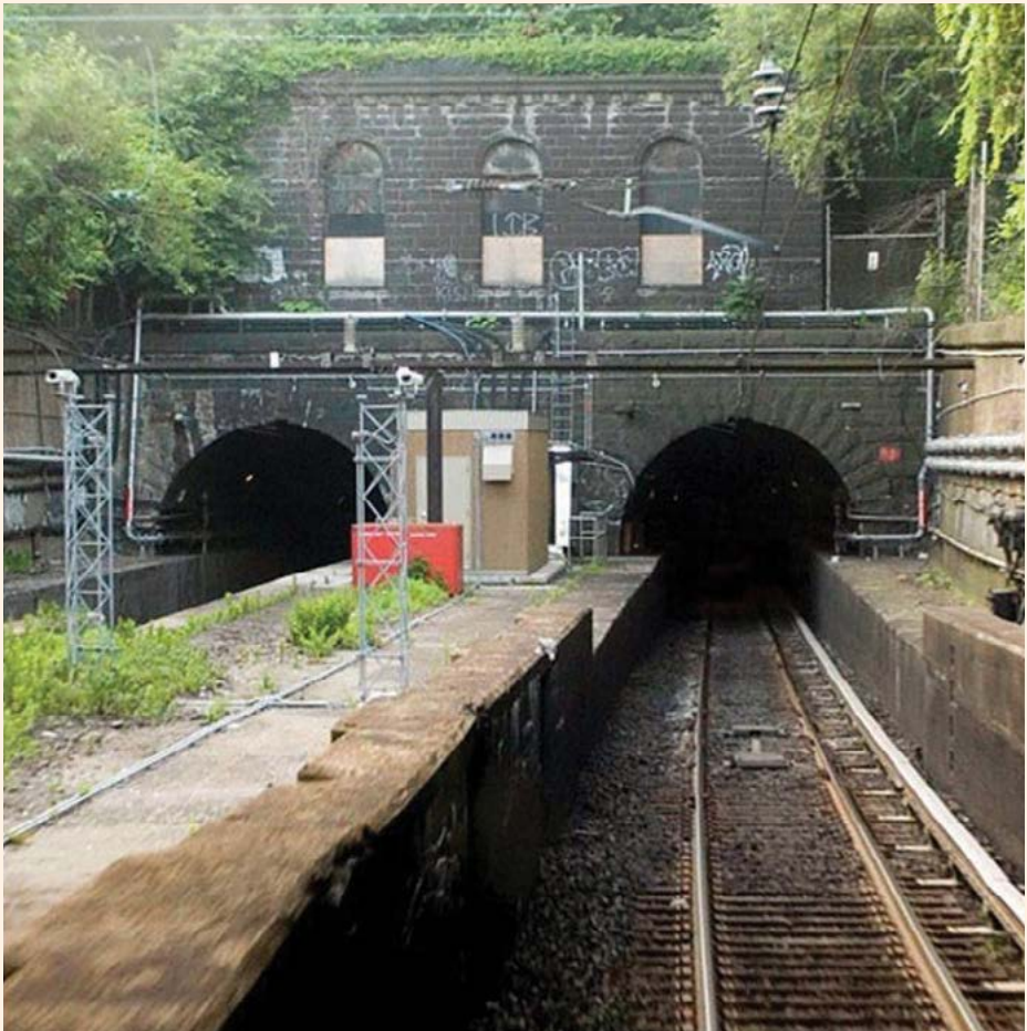
Figure 42 Trans-Hudson Tunnels, linking New Jersey and New York
