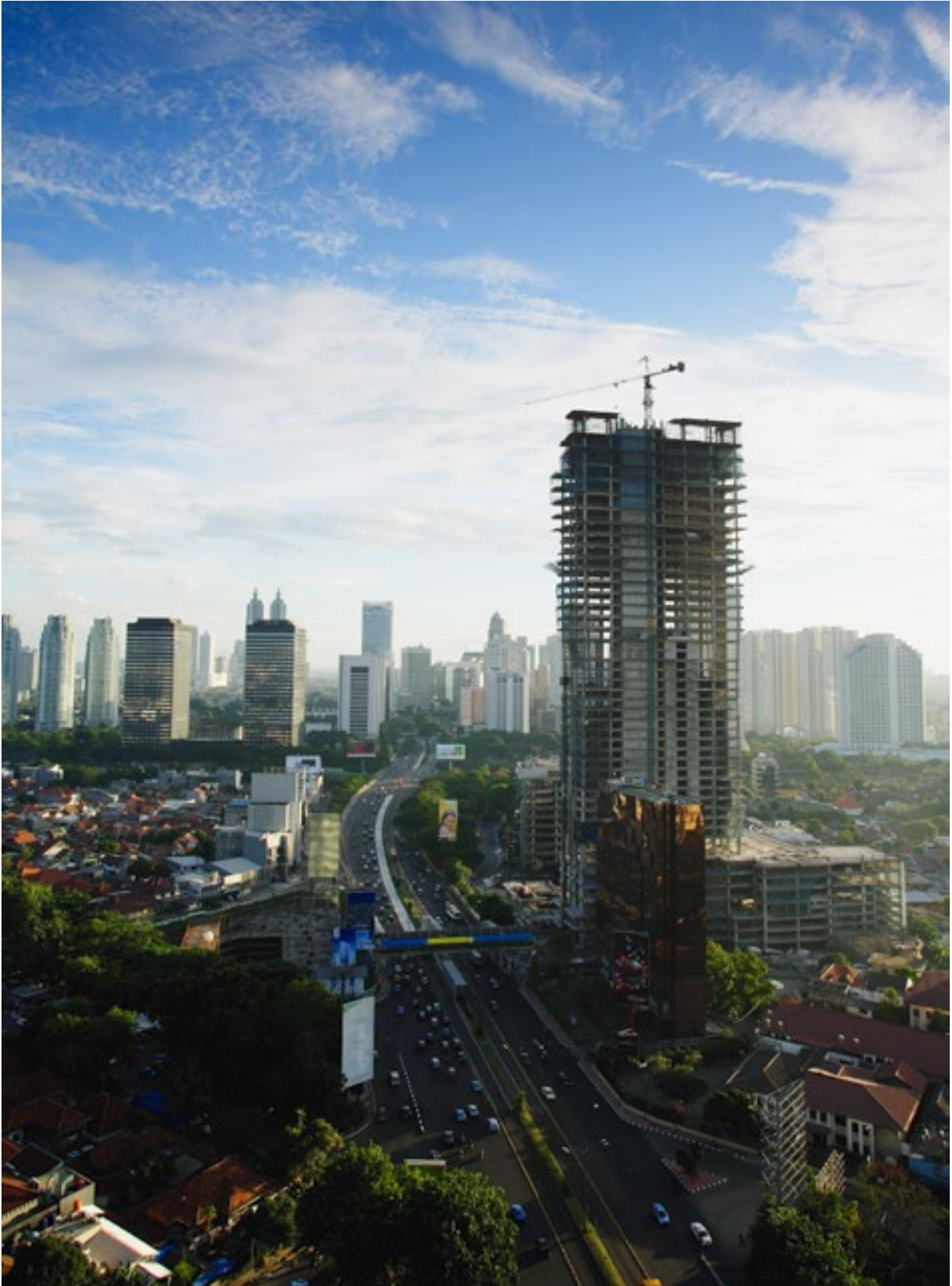
Late afternoon view of the CBD with building construction and office skyscrapers along Jalan Jend Sudirman, Jakarta © Martin Westlake/Asia Images/Corbis.
