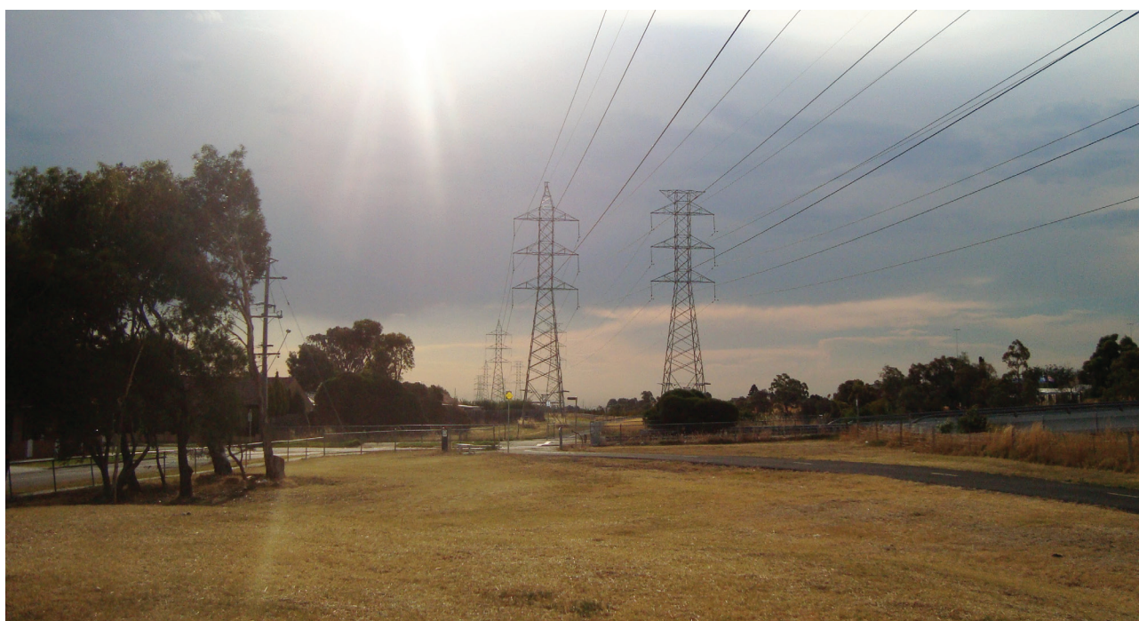
Figure 9: Electricity pylons during a heatwave; extreme heat puts increasing pressure on infrastructure.
