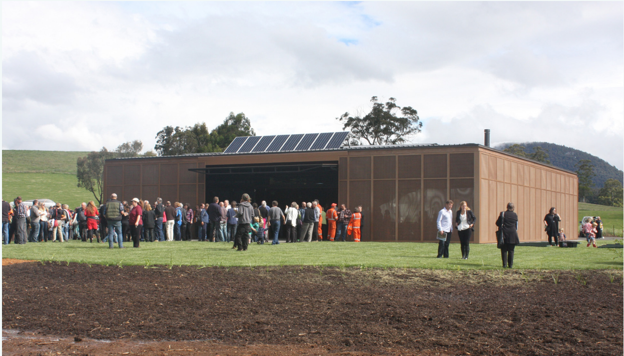
Figure 4. Narbethong Hall on its opening day. (Picture reproduced courtesy of ARUP)
