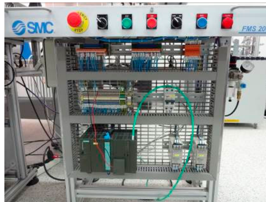
Figure 2. Front panel and keypad of one of the stations.
