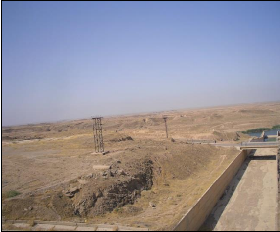
Picture 5.1: The Udham Dam spillway. Taken on 09.03.2014
