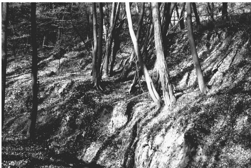
Figure 10.12.: Younger landslide area within the landslide complex ‘me5’. Note the tilted trees and the coupling with the stream (in foreground). (photo: Volkhard Schmanke)
