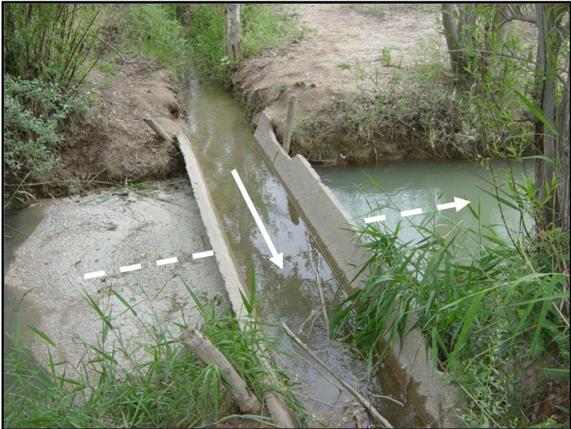
Figure 7.2 – Crossing ditches; one with pumped water and one with gravity water
