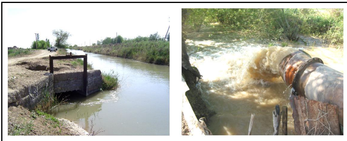
Figure 5.9 – Gravity and pumped off-take from main R8 system to WUAs
