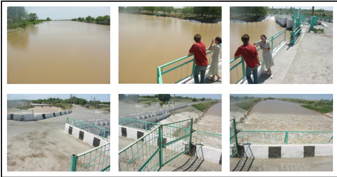
Figure 5.3 – Tashsaka Zaruzenya one of the main division points operated by UPRA DIK. The inflowing canal has a design capacity of about 500 m 3 /s (1st till 3rd picture) and splits into canals with capacities of about 250 m 3 /s (4th picture) and 200 m 3 /s (5th and 6th picture) plus a few smaller ones. The pictures were taken by Jan Sendzimir
