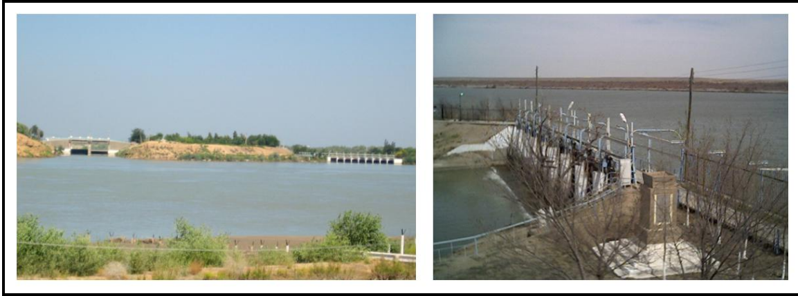
Figure 5.2 – One of the river off-takes (at Tashsaka) operated by UPRA DIK
