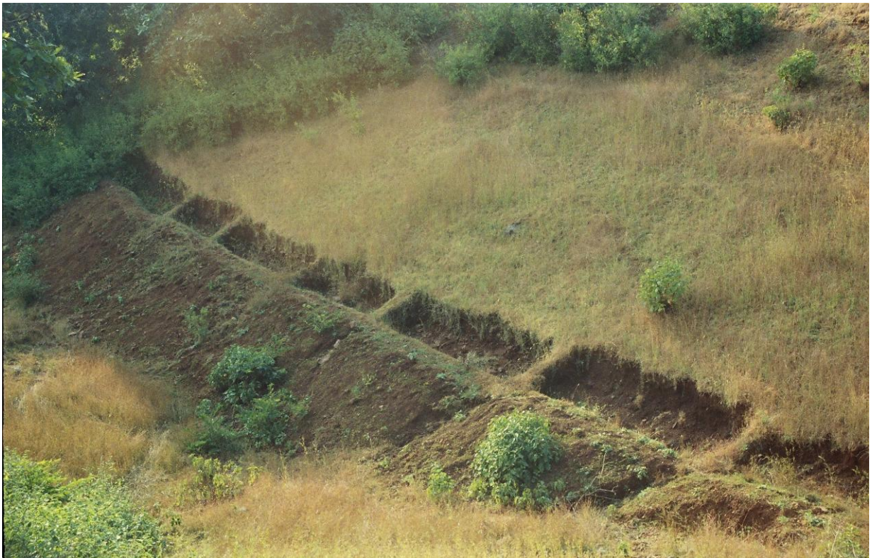
Photograph 1. Continuous Contour trenches in Pimpri Village
