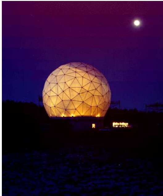
Figure 4.1: The FCRAO 14-m telescope dome near Amherst. The telescope is enclosed in a radome structure.
