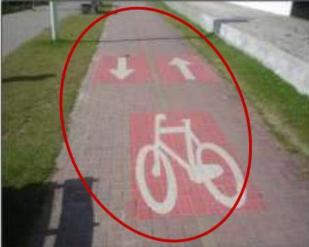
**Figura 36 – Piso de pavers.**
