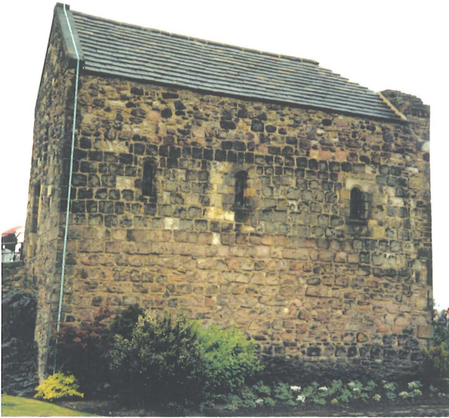
Figure 96 Exterior view of St Margaret's Chapel, Edinburgh Castle, c.1100
