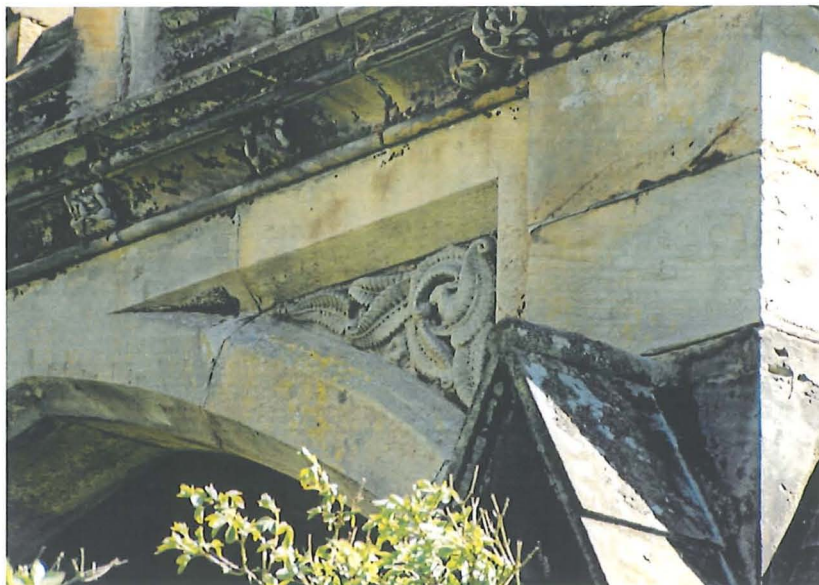
Figure 8 Detail of entrance porch, Crawford Priory, c.1870
