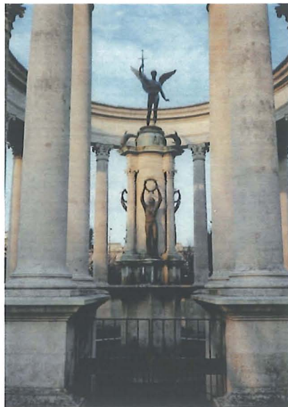
Figure 95 Detail of central podium and seating: Welsh National War Memorial, Sir J. Ninian Comper, 1924-28
