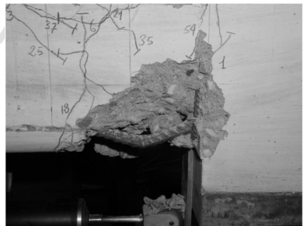
Fig. 11. Specimen REF100: buckling of a longitudinal bar at a critical region.
