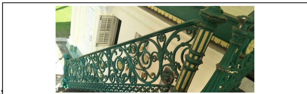
Figure 6: Image of The Cast Iron Balustrade at Staircase
