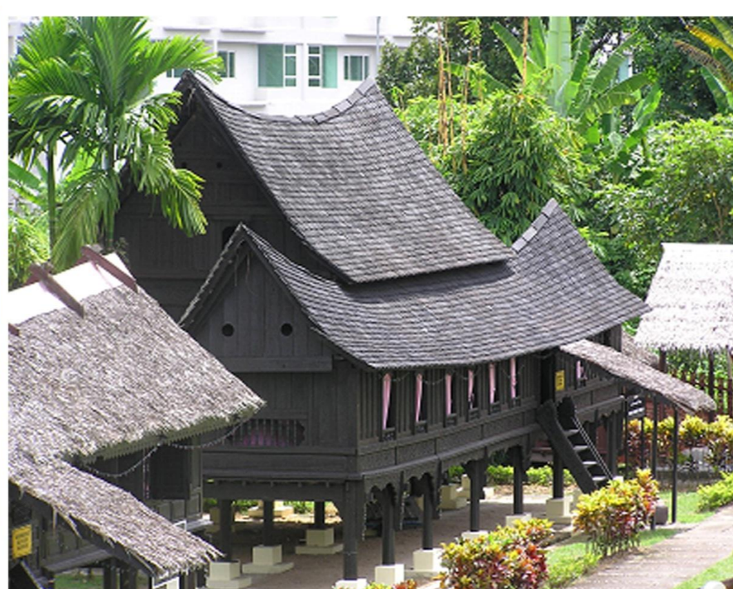
Minangkabau houses on display in Negeri Sembilan: the right building uses timber tiles for the roof whilst the left building uses traditional thatch roof.
