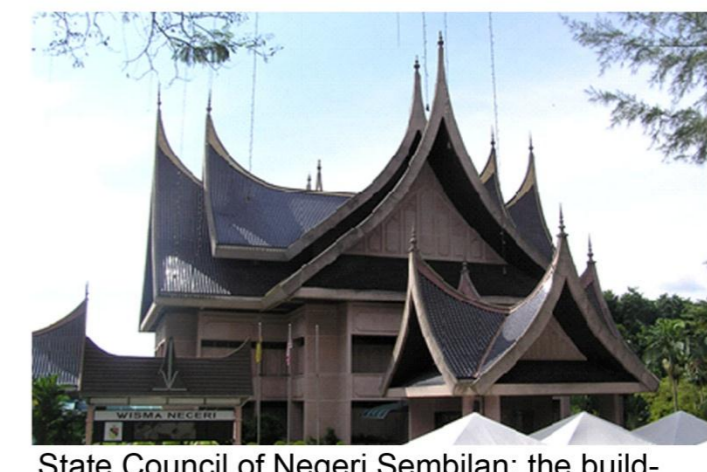
State Council of Negeri Sembilan; the building was constructed using modern construction method and materials.
