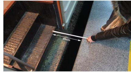
Fig.4. The unsafe gap in the Vukov Spomenik railway station in downtown Belgrade
