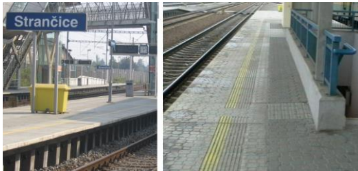
Fig.2. SUDOP type platform (left) and tactile ground surface (right)
