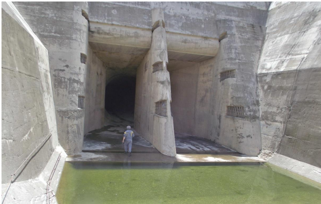
Figure 2. FP-BA tunnel entrance building
