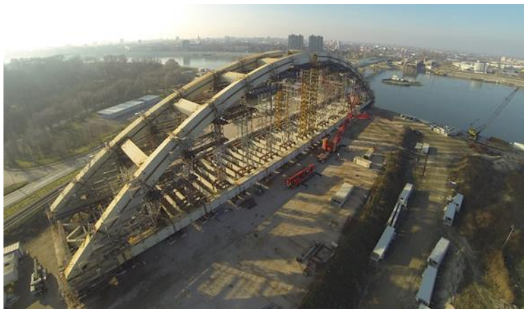
Fig. 14: Aerial view of the site. Arch 177 m, Jan. 2014
