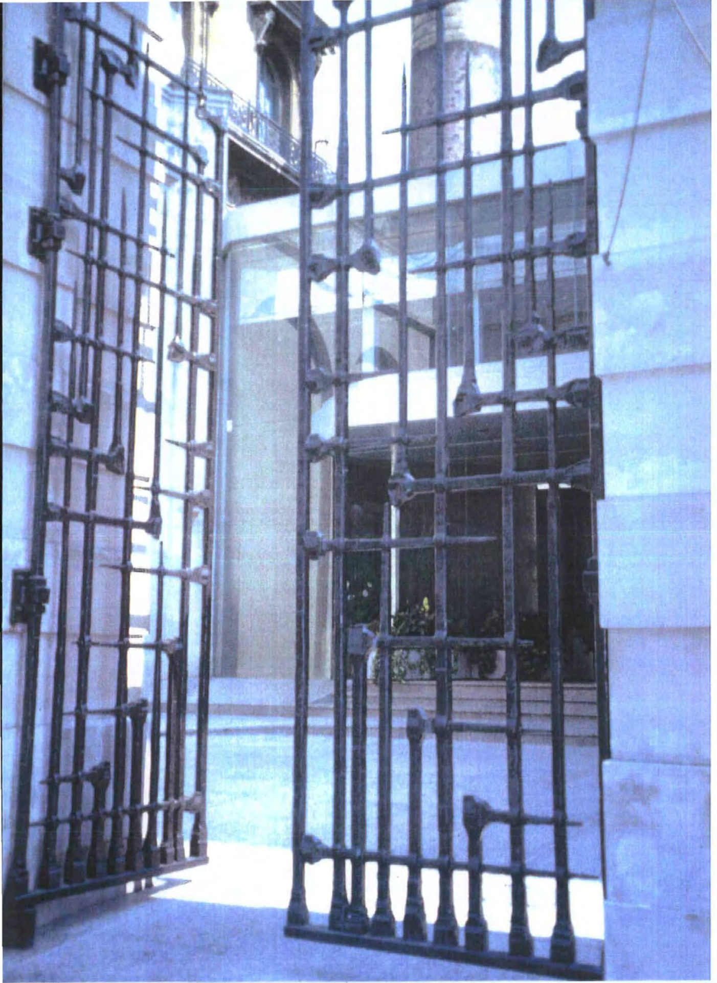
Figure 48. Site photograph, Giuseppe Lund's Victoria Plaza gates, 1985, forged and fabricated mild steel.
