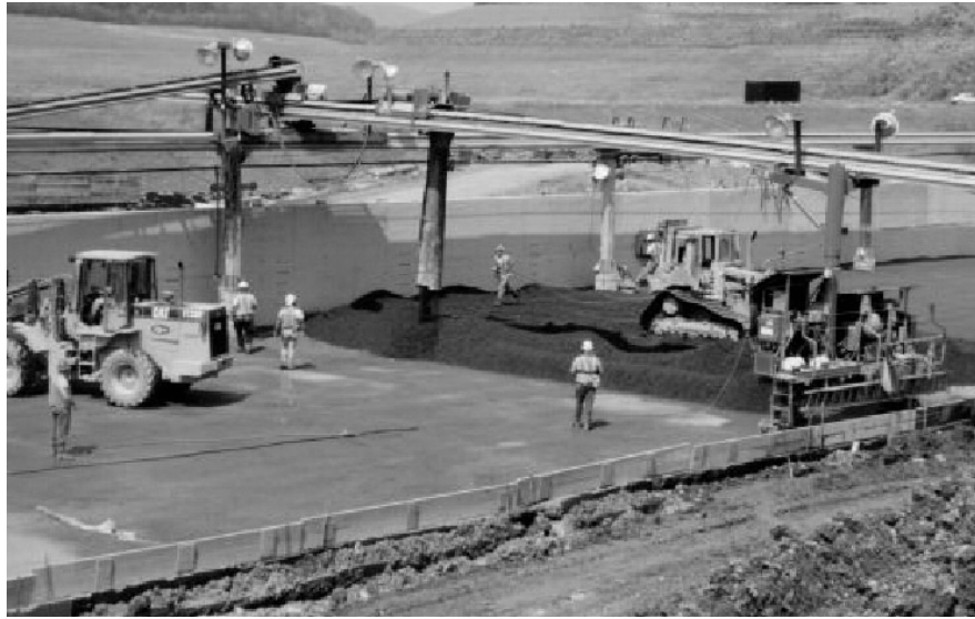
Figure 3.5: Transporting RCC by conveyor belt.
