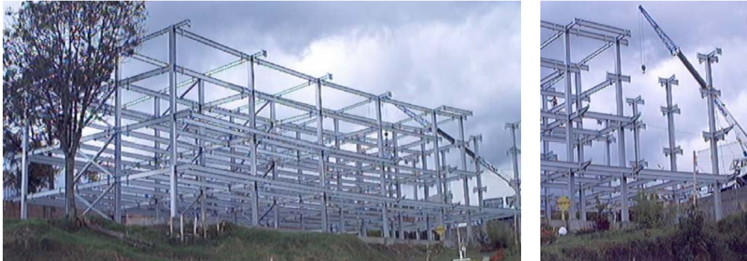
Figure 5. Building under construction.
