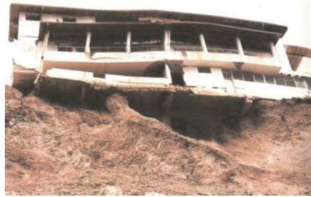
Figure 4. Ground conditions, landslides and ground failure.
