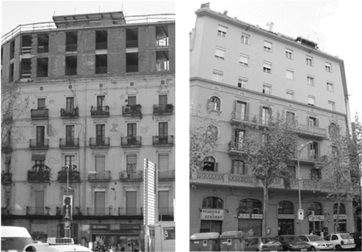
Figure 1. Example of URM buildings with high seismic vulnerability. The addition of top levels to the original buildings increases even more their seismic vulnerability.
