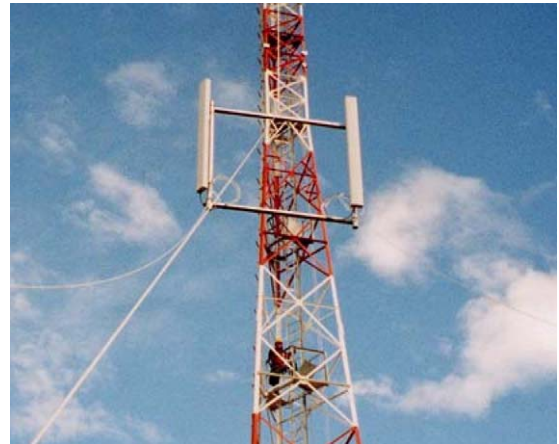
Fig. 17. Base station panel antennas being installed at Los Leones.
