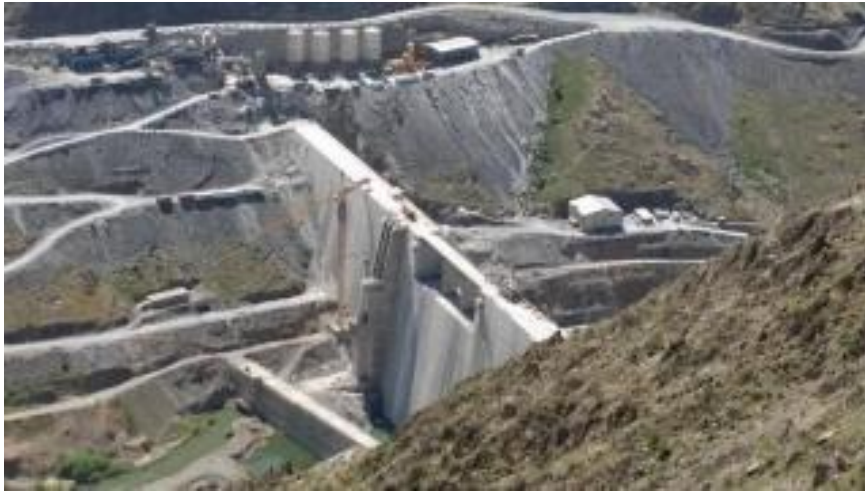
Figure 5: Dam construction in Sanandaj, Source: Azizi, 2019
