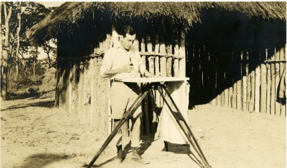
Fig. 7. Cuthbertson in the bush using a plane table for surveying, 1930. Photograph courtesy of the Smithsonian, Washington, DC.
