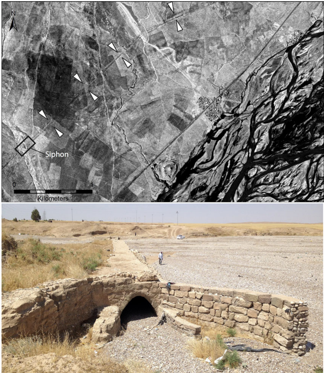
Fig. 11 1969 CORONA satellite image revealing a major likely Sasanian canal west of modern Kalar (top). Several stone built siphons are preserved where the canal once crossed seasonal drainages, including this partially reconstructed example (bottom)
