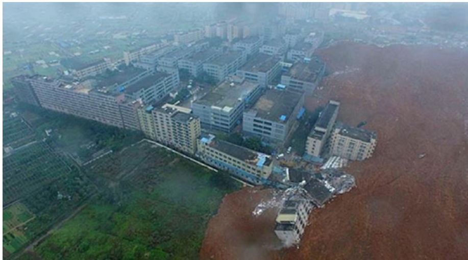
Figure 2.5: C&D waste landfill landslide in Shenzhen, China [51].
