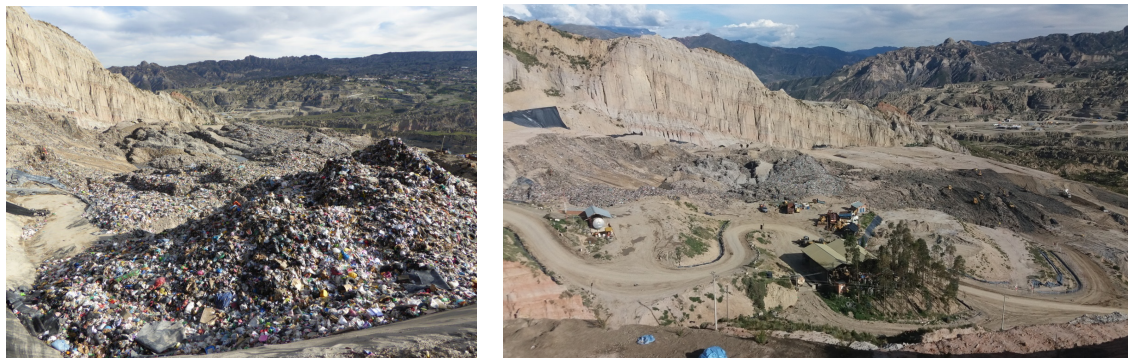
Figure 2.15: Collapse of the sanitary landfill in January 2019. Photos took at the end of January 2019 during a technical visit at the final disposal site.
