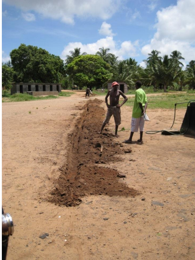
Photo 13 Community contributes to digging a piped scheme, Mozambique.
