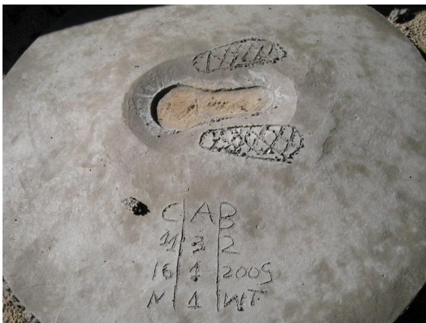
Photo 2 A slab for a latrine in Mozambique.
