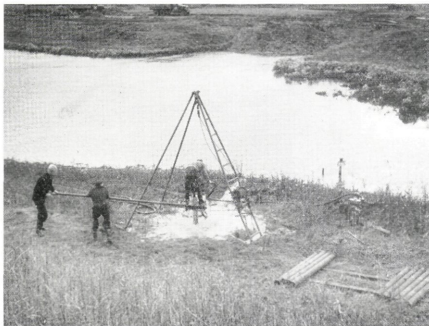
Fig. 2.—Wash boring to a depth of 40 m. carried out just behind the sea dike. The observations from this well are used to study the transmission of the tidal wave in the artesian basin
