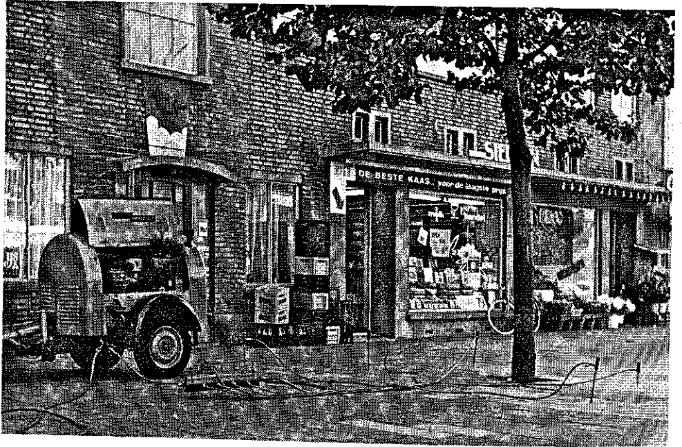
Fig. 32. Compressor treatment near a tree affected by gas leakage (photograph VEG-Gasinstituut, Rijswijk).
