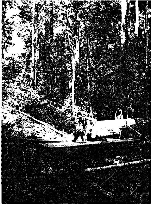
FIG. 152. Local people, transforming logs into beams by hand.
