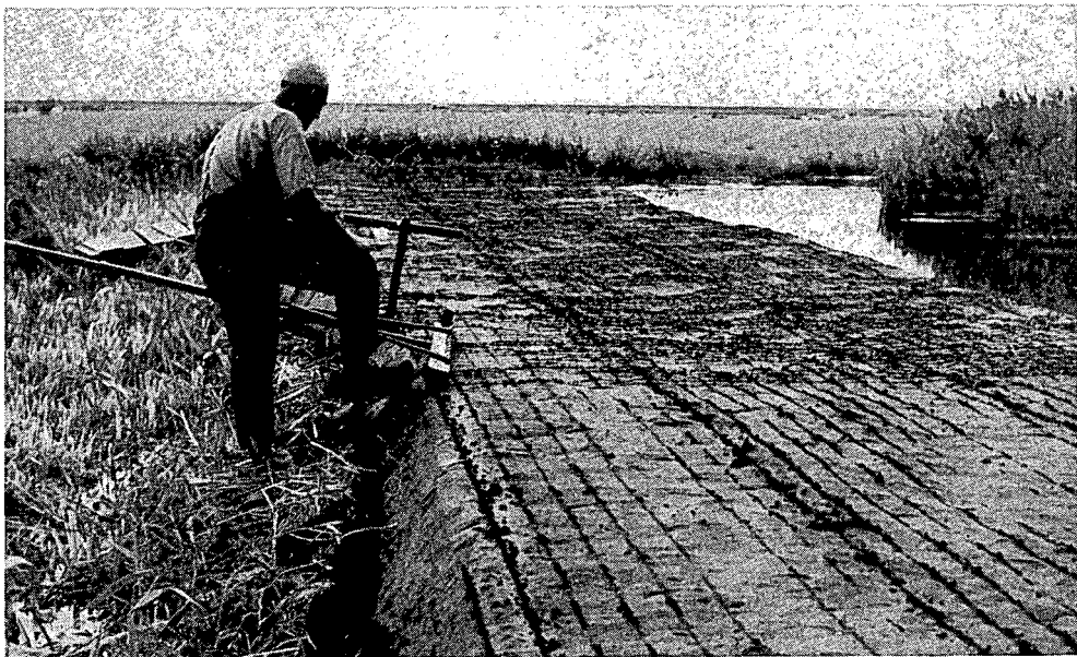
Figure 3 Some days after dredging the peat, the partly dried sludge is scratched with a rake to indicate the size of the blocks to be cut after further drying (Photo Soil Survey Institute 22405).
