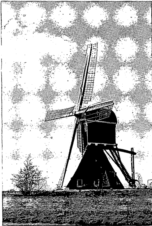
Figure 2 Windmill formerly draining a peat-polder area West of Utrecht (Photo Soil Survey Institute R 31-155).
