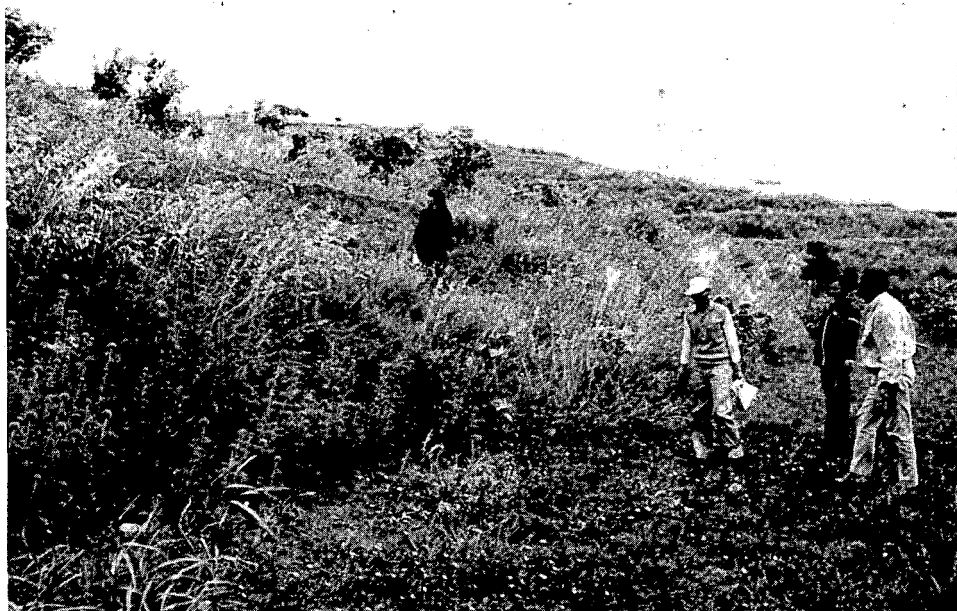
Figure 18.10 Landslide in the riser of a large bench terrace on heavy clay. The Vertic properties of the clay cause instability of the risers in the moist winter season. Steep risers accompanied by large step heights cause this phenomenon.
