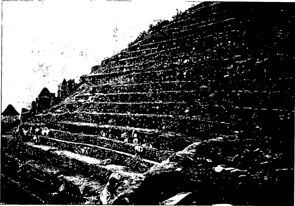
Figure 4.2 Stone terraces at Machu Pichu, built by the Incas more than 400 years ago. The tallest terrace wall measured was 7m high.
