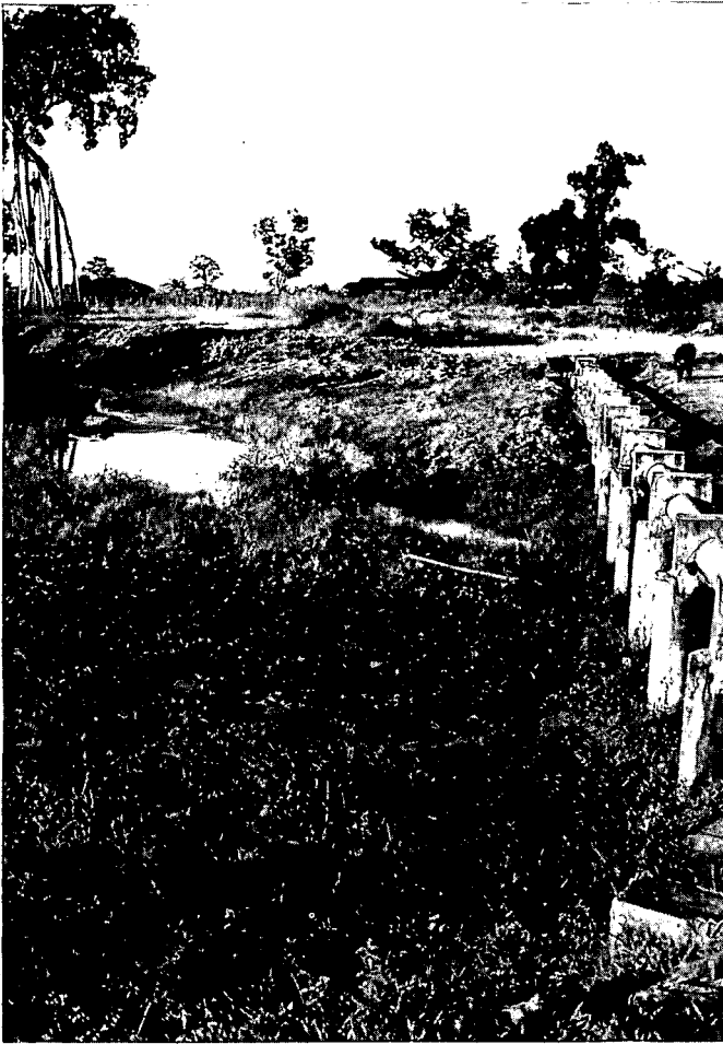
Photo 5.1 A leaking concrete irrigation pipe crossing a major drain perpetuates breeding places for mosquitoes
