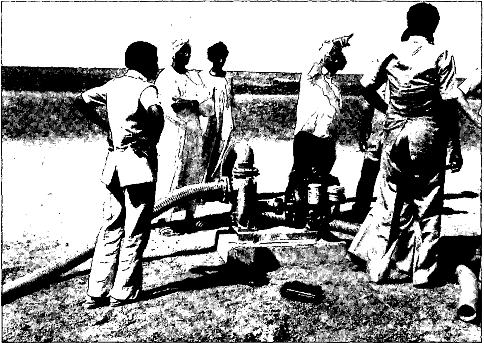
Figure 4.9 Village drainage pumps installed during malaria transmission season.
