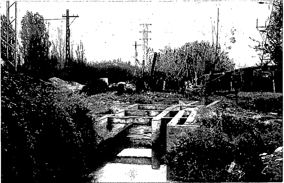
Photo 1 Proportional divisor with fixed pier in between the two weirs
