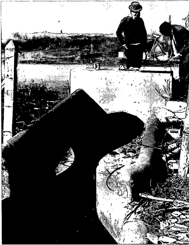
Photo 2 Throatless flume with rounded transition
