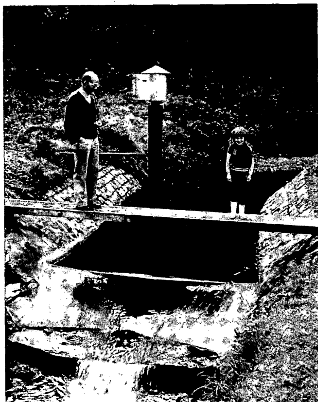
Photo 6.1 An 1-to-2/1-to-5 shaped weir on a natural stream
