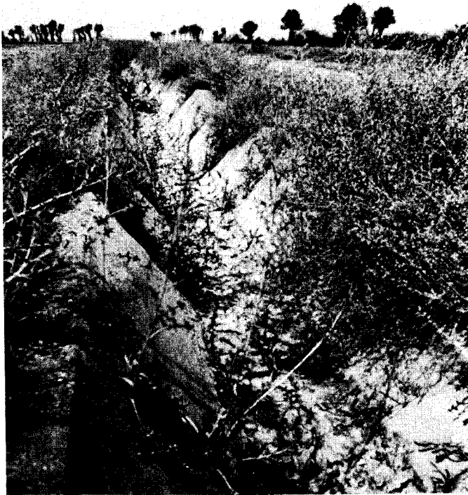
Photo 3 and 4 If structures and lined canals are not properly maintained, they will contribute little to the efficient use of irrigation water
