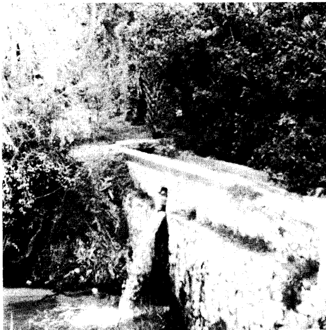
Photo 2 Water flowing from an irrigation canal straight into a drain adds to the 'management losses'
