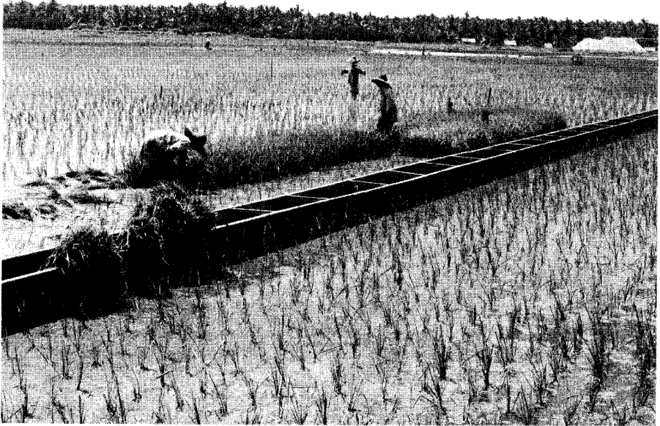
Photo 10 Properly levelled fields, a lined distribution system, and skilful operation and management of the irrigation system ensure a high efficiency of water use
